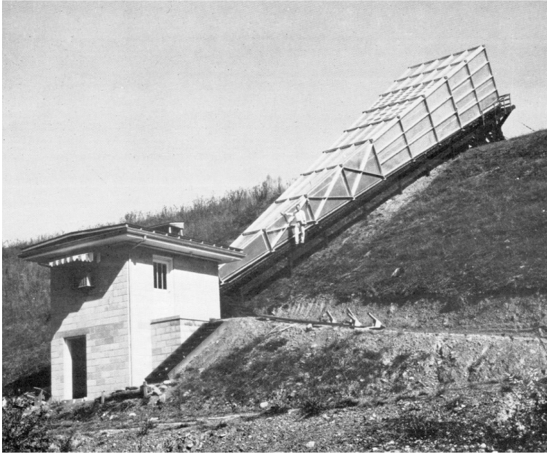
Figure 6. The Little Big Horn at the NRAO, Green Bank. The aperture was 5.4 m × 4.0 m, and the length was about 36 m. Cas A crosses the beam daily, and a measurement of its flux density is made at 1440 MHz (NRAO/AUI/NSF).
